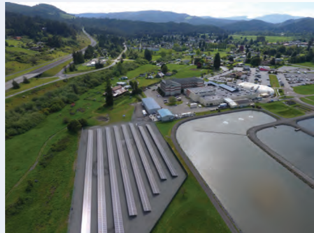
Aerial view of the Blue Lake Rancheria 500kW solar array within the Tribe's low-carbon community microgrid (Photo: Blue Lake Rancheria)
